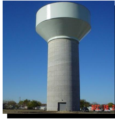
Water Delivery System Development
